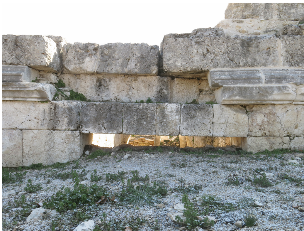
Fig. 16a: The southern straight arch door of stage building
