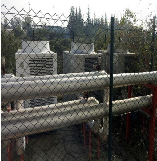
Akdeniz University, Athletics Stand (Stadium) Air-to-Water Heat Pumps on the East and West sides.
