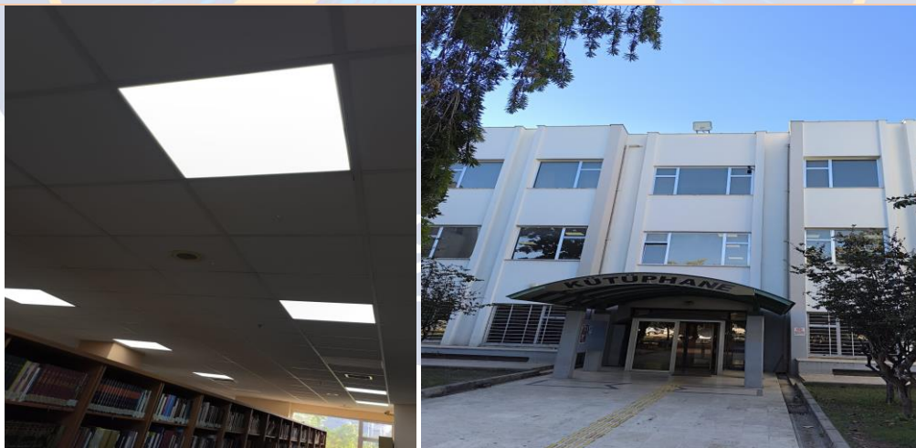
Example of Energy-Efficient Device Usage: The Use of 60x60 cm 36W LED Panels and LED Outdoor Lighting Projectors at Akdeniz University
