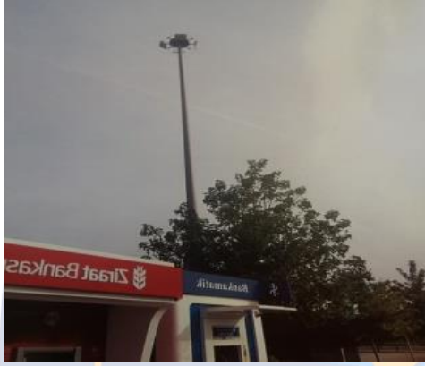
Solar street lamps
