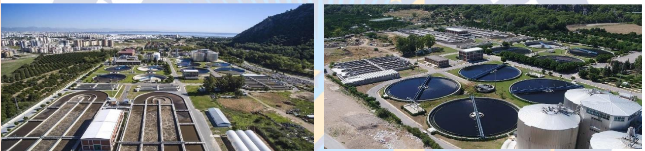
Hurma Wastewater Treatment Plant
